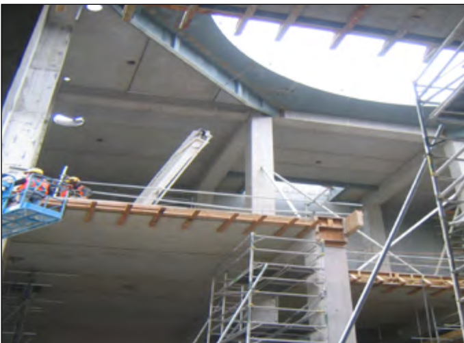
Steel roof structure
