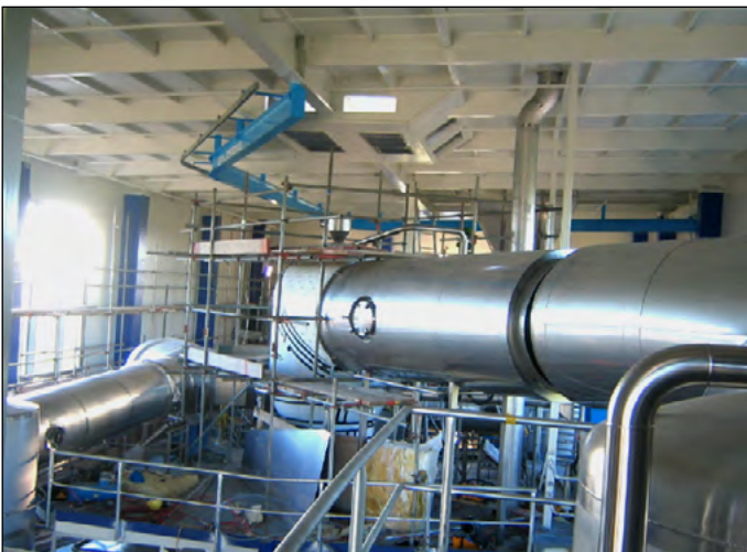
Steel roof structure
