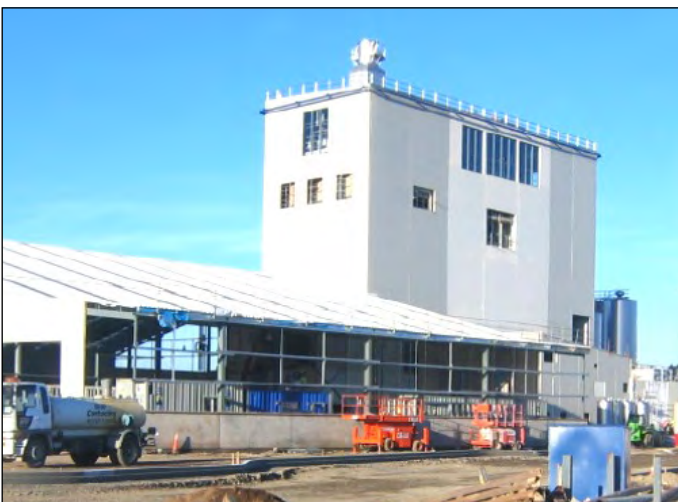
Chevaline Colourglaze to exterior walls
