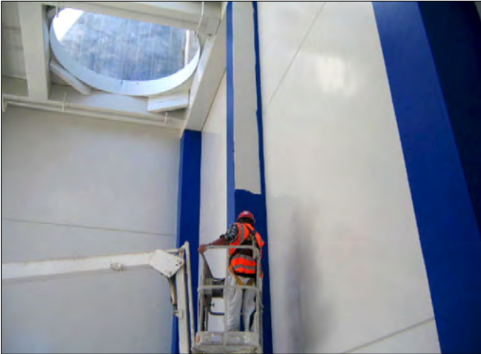
Chevaline Colourglaze to interior walls
