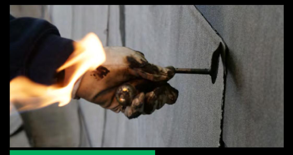
EQUUS SOPREMA COLPHENE BSW TANKING SYSTEM
