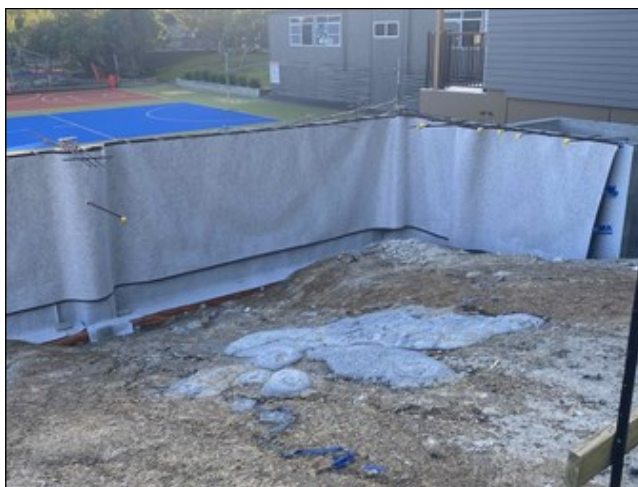
Installation of Equus drainage, filter and protection layer
