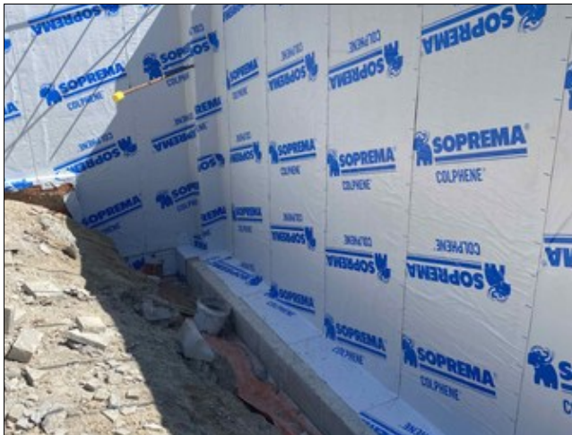
Completed wall waterproofing
