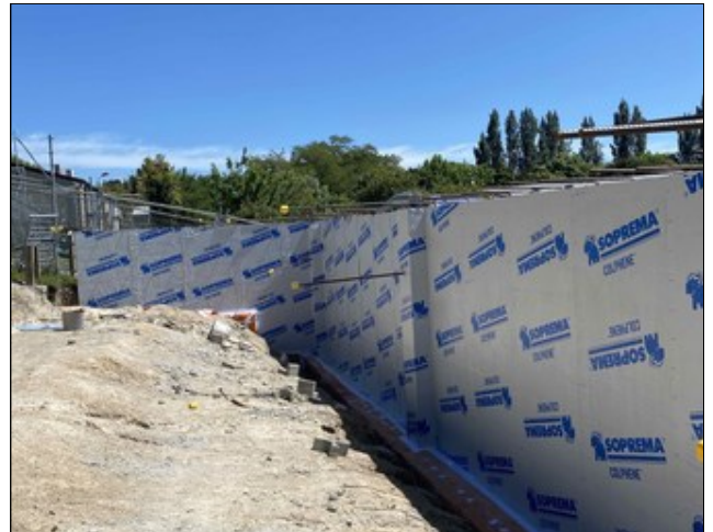
Connection of COLPHENE 3000 waterproofing membrane to DPM
