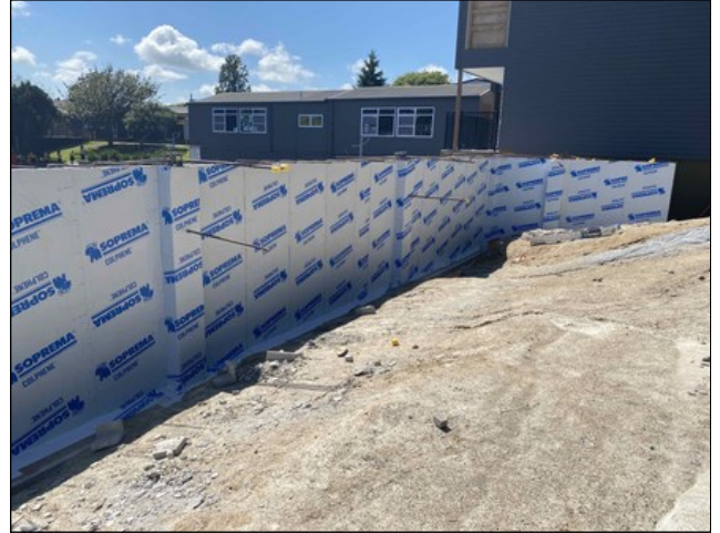
Installation of COLPHENE 3000 below-ground waterproofing
