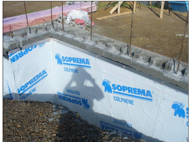
COLPHENE 3000 waterproofing membrane to wall
