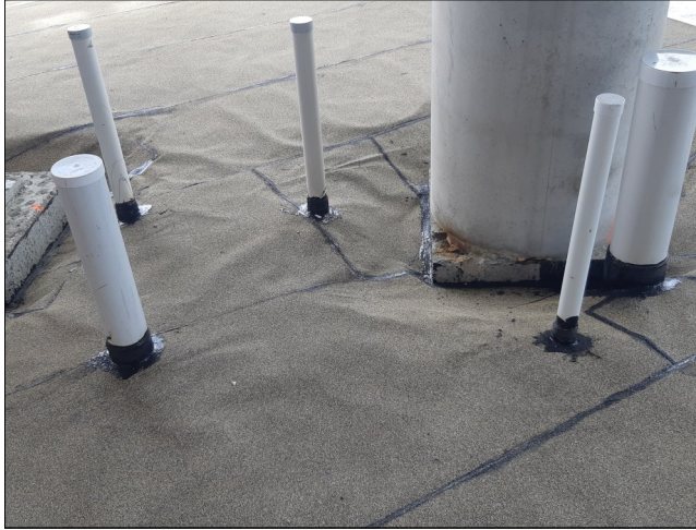
Pipe penetration detailed with Liquid applied membrane
