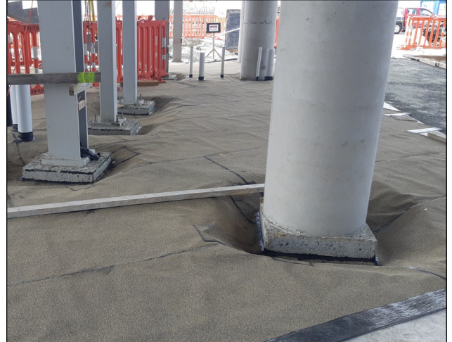
Flexibility of the membrane helping the DeboFlex conform to the substrate
