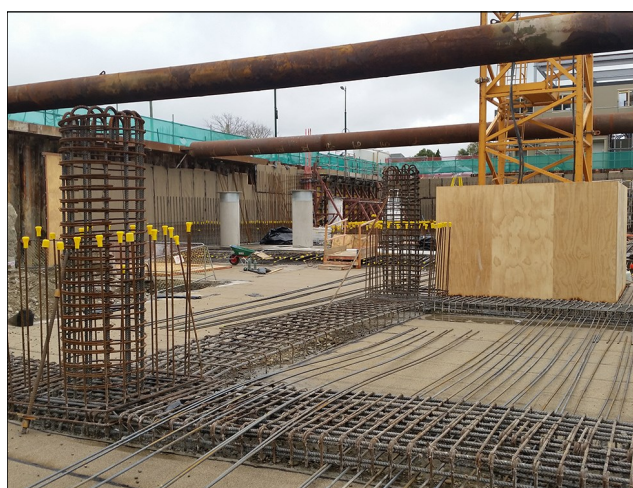
Reinforcing steel installation
