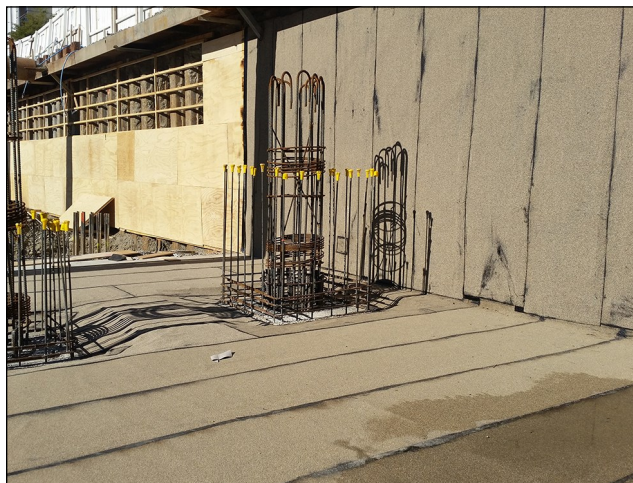
DeboFlex 3.5 Special dressed into pile caps
