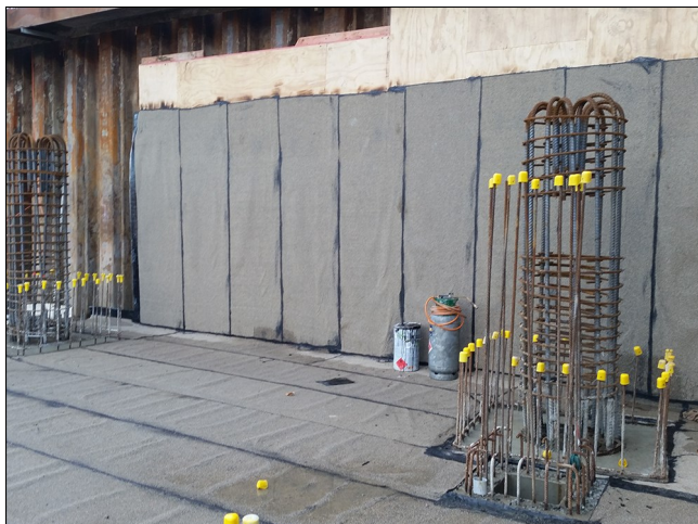
DeboFlex 3.5 Special to concrete slab and timber lost formwork
