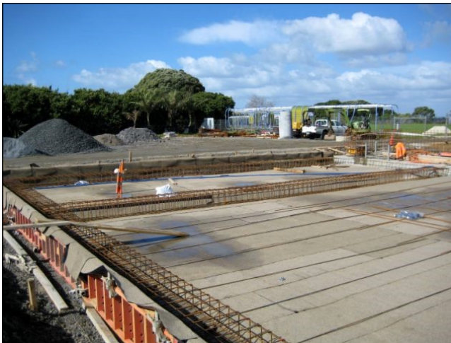
Steelwork installation over Debobase
