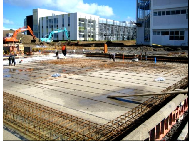
Steelwork installation
