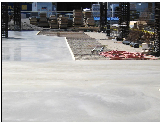
Completed tanking and concrete pour
