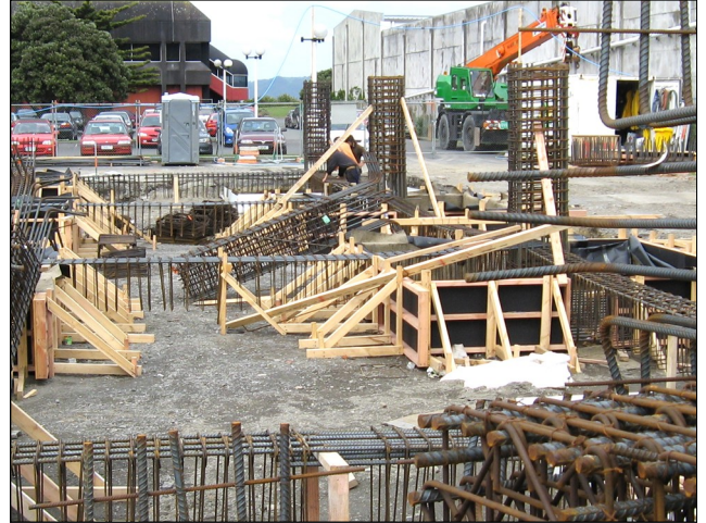
Prepared site ready for tanking installation
