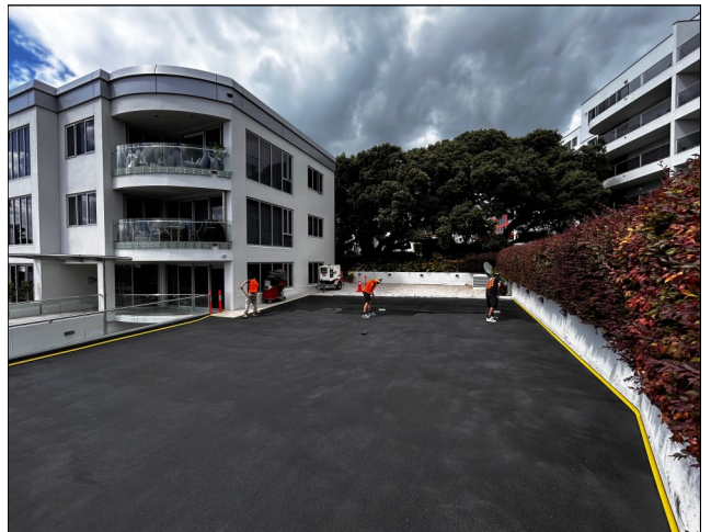
Second and final application of Matacril STC (Clear) Topcoat
