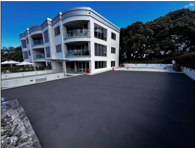
Matacril 215 Wear layer is broadcast with charcoal aggregate
