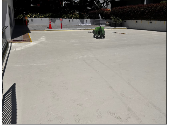
Matacril waterproofing layer applied
