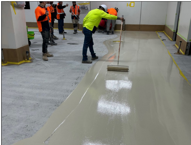
First layer of body coat
