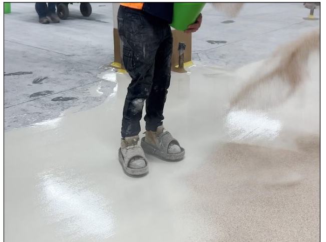
Broadcasting the aggregate onto the body coat
