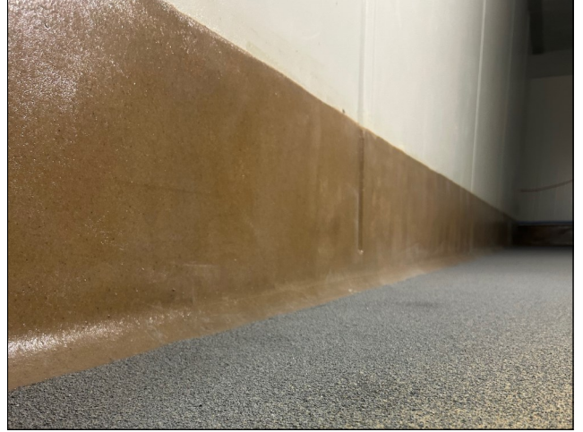
Epoxy cove installation
