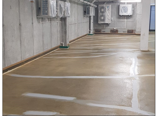
Matacryn LM used to fill cracks after priming
