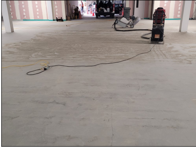
Substrate prepared with grinding
