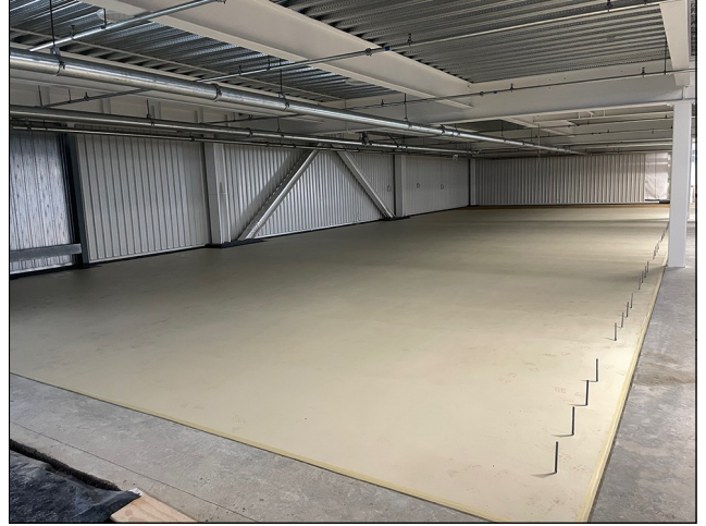
Matacryn Manual membrane layer laid
