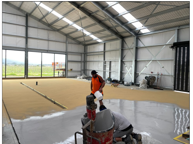
Broadcasting the aggregate onto the body coat
