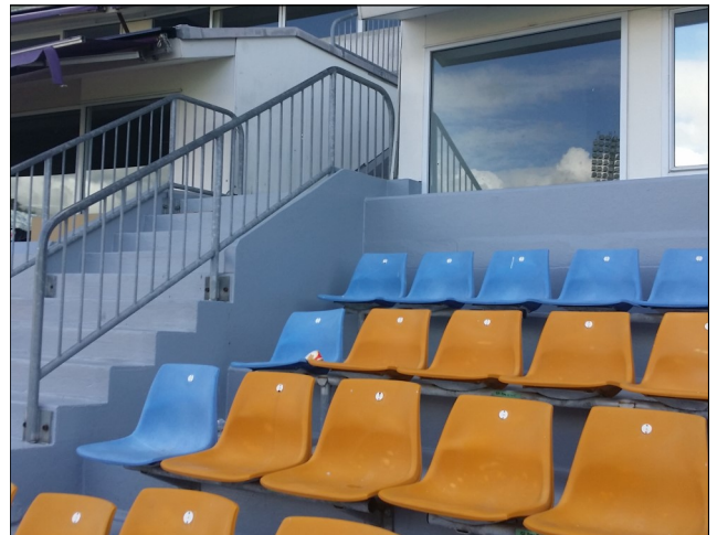
Matacryn Membrane applied to stairs and aisles
