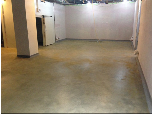
Primed concrete substrate
