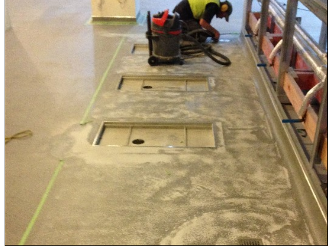
Preparation of substrate
