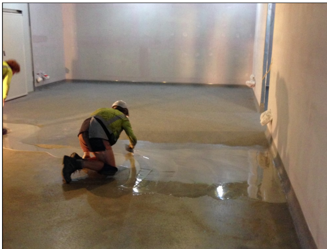
Application of Duracon BC wearcoat
