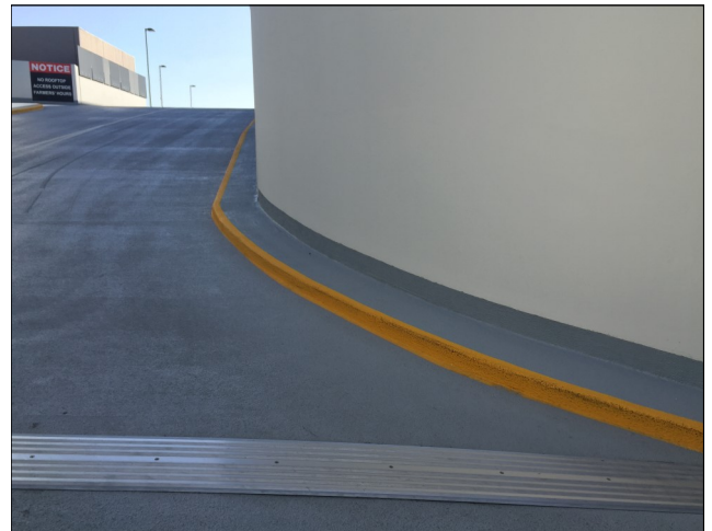
Completed Matacryn Carpark to ramp
