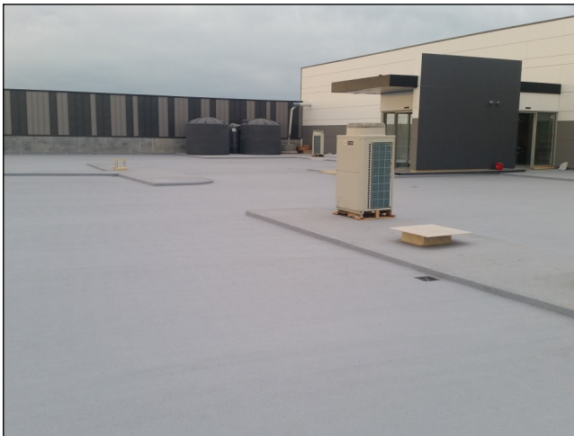
Application of Matacryn carpark membrane
