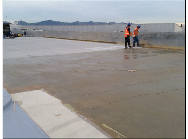
Primer Application to concrete substrate
