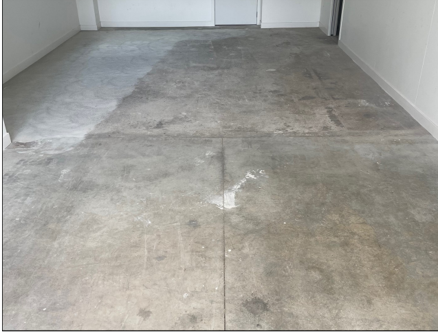
Existing garage floor
