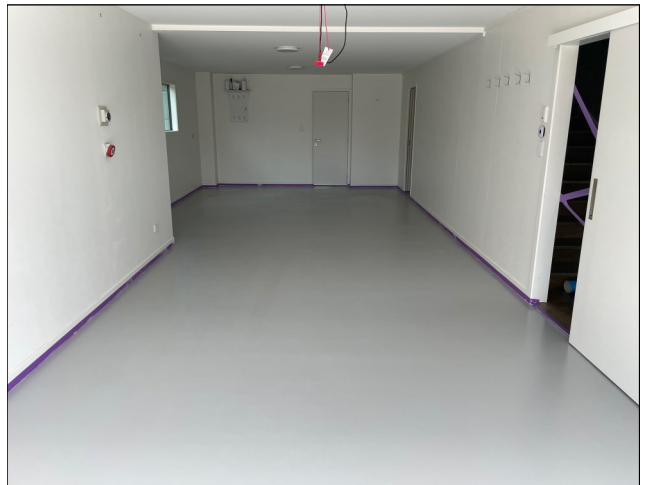
Epistixx Rapid Topcoat applied over Epistixx primer
