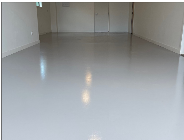
Additional coat of Epistixx Rapid Topcoat applied to complete the project
