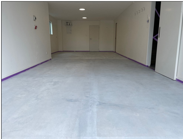
Epistixx primer applied to existing concrete
