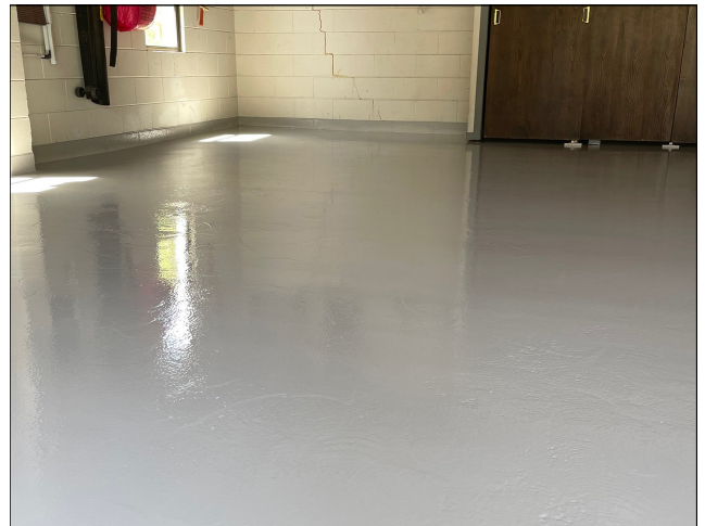
Epistix Rapid 3x coat system applied to concrete
