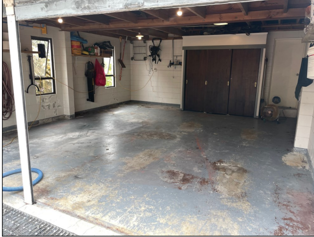
Existing garage floor
