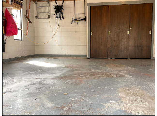
Existing coating lifting due to wear from car tyres
