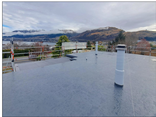
Installation of Flagon TPO waterproofing
