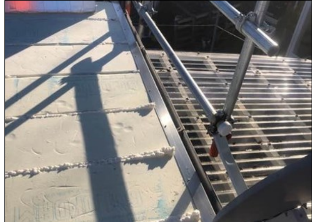
Installation of XPS infills glued between the metal ribs to provide a base for the PIR to be installed
