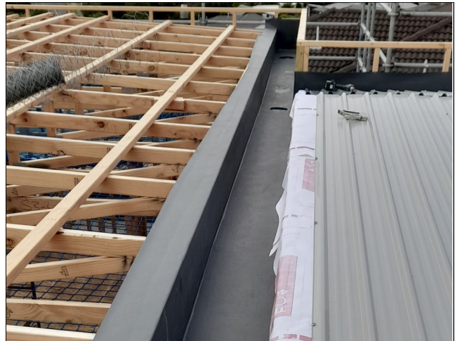
The FLAGON TPO membrane provides a smooth and aesthetic finish for internal gutters
