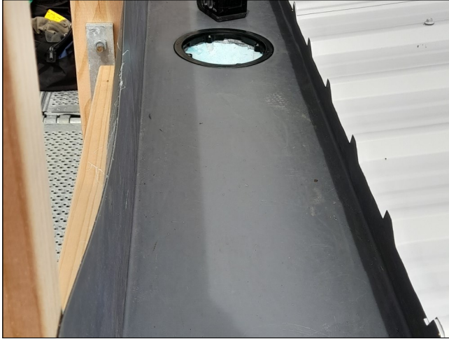
FLAGON TPO membrane into gutter by fully adhered, flameless installation
