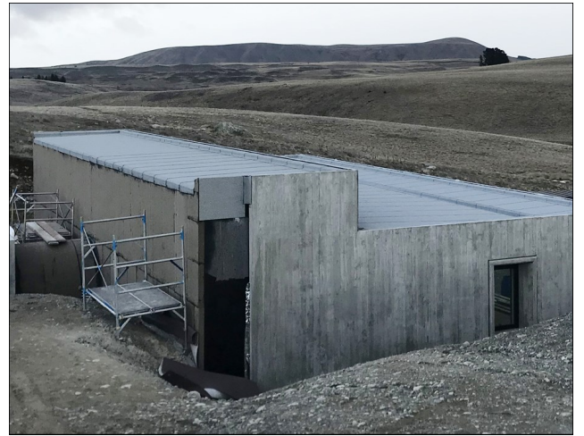
Cap sheet completed
