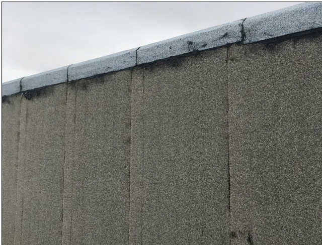
Cap sheet connection to wall tanking membrane
