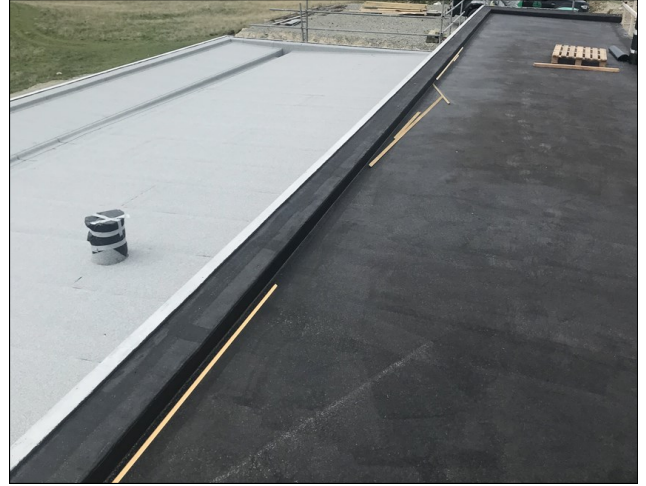
Installation of primer on top roof
