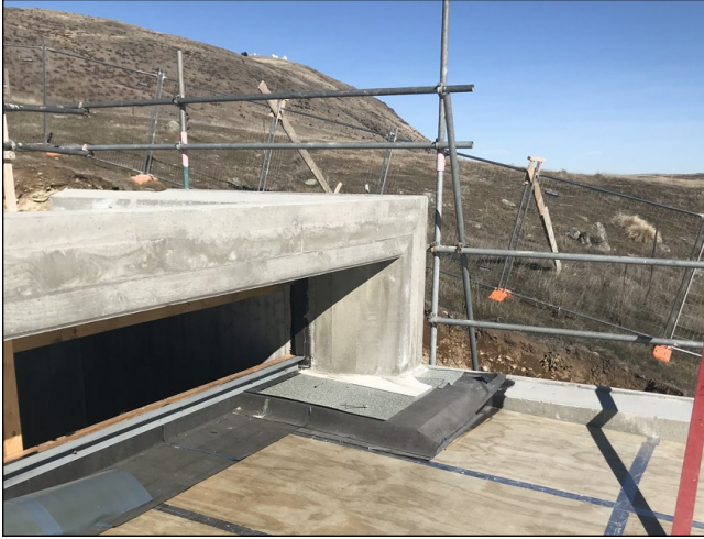
Installation of substrate
