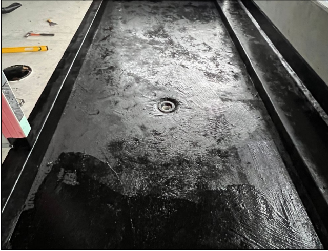
Application of SOPRADERE QUICK primer
