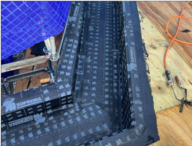
Installation of SOPRSUN PLUS 3 base sheet
