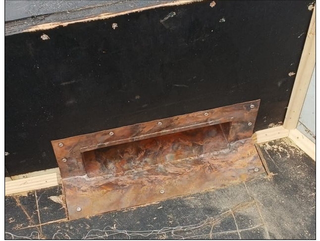
Installation of copper scupper drain
