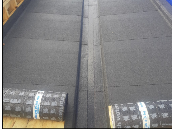
Installation of SOPRASUN PLUS MINERAL cap sheet
