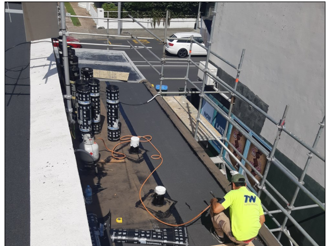
Cap sheet being torched to base sheet
