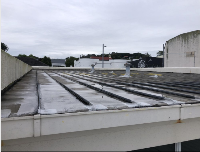
Original iron roof
