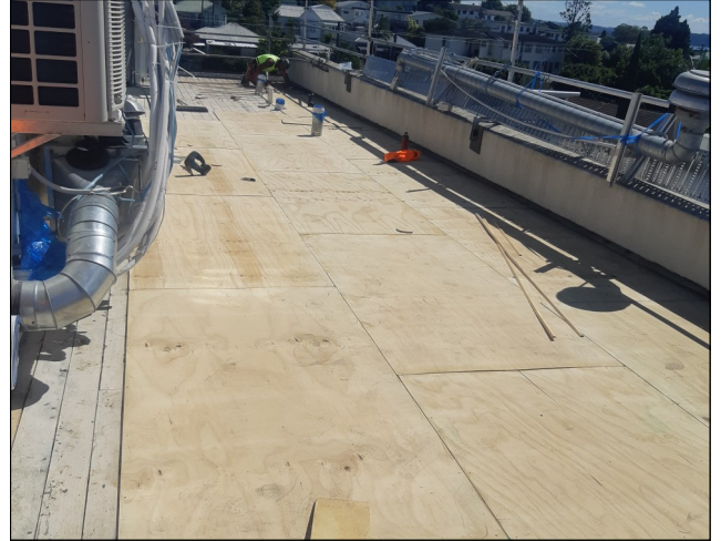
New ply on existing sarking timber
