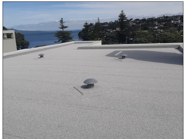
DUO cap sheet torched on over base sheet
