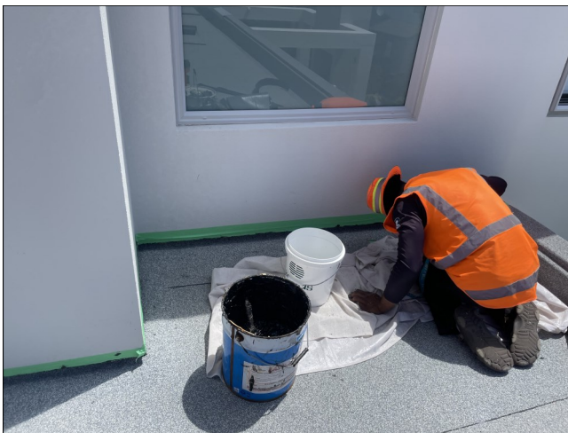
Under the cladding SOPREMA EASY FLASHING is used
