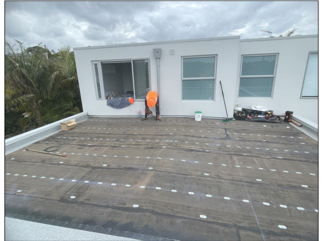
Base sheet mechanically fastened over existing membrane
