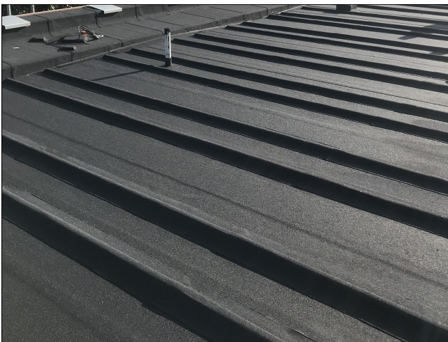
DuO AGR (Black) Cap Sheet and solar panel plinths installed
