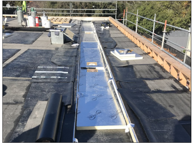
Thermal insulation installed under base sheet
