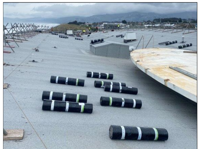
Installation of DUO cap sheet
