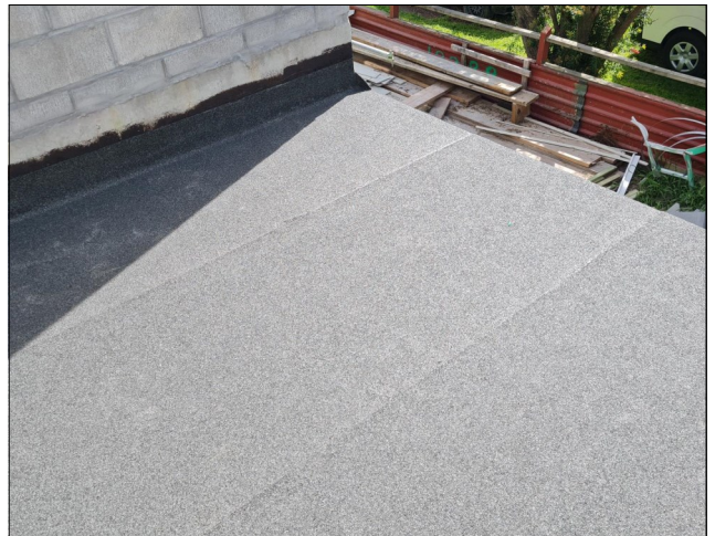
Easy malleable APP membranes available in torch applied and self adhered
