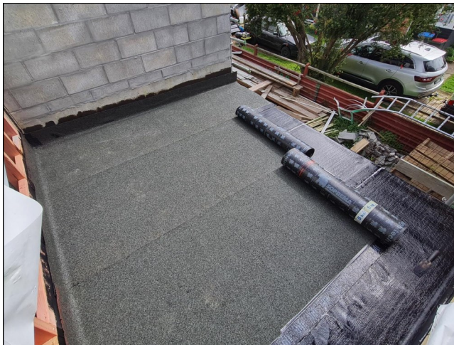
Polibit Mineral dark grey cap sheet being applied
