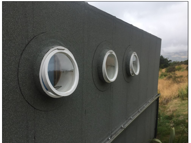
Completing detailing on windows
