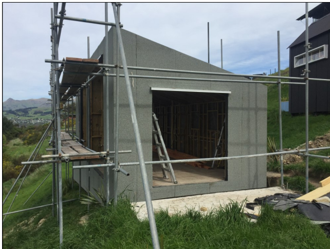
Finishing walls and detailing thresholds
