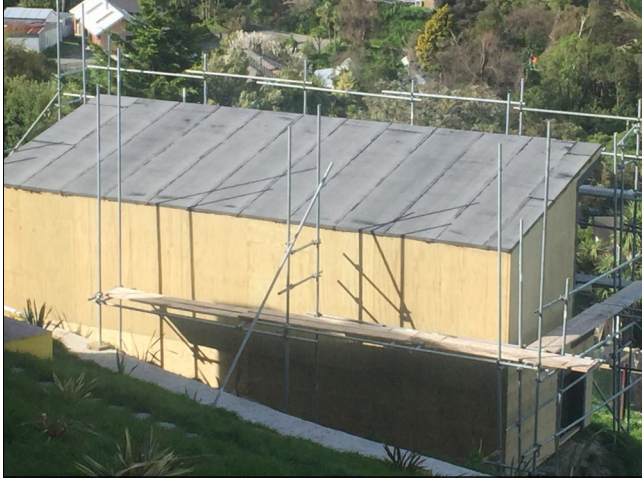
2.5mm DeboFlex base sheet of roof being installed
