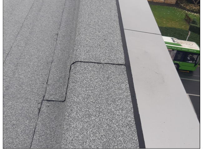
Alsanc Mastic 2200 sealant to seal DuO capsheet against aluminium parapet capping
