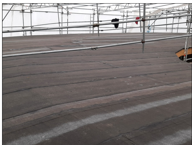
DeboPlast base sheet being applied
