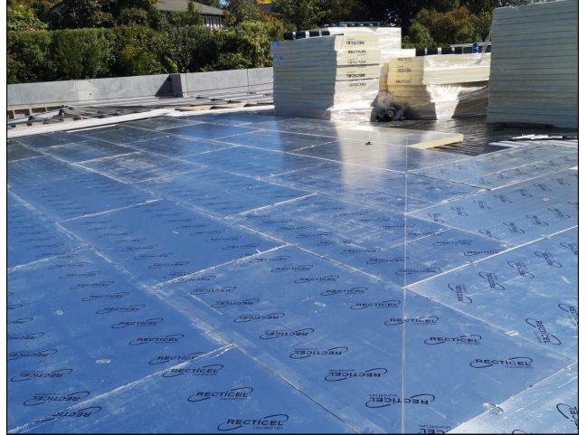
Installation of vapour barrier and thermal PIR insulation
