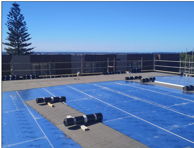
Installation of waterproofing base sheet
