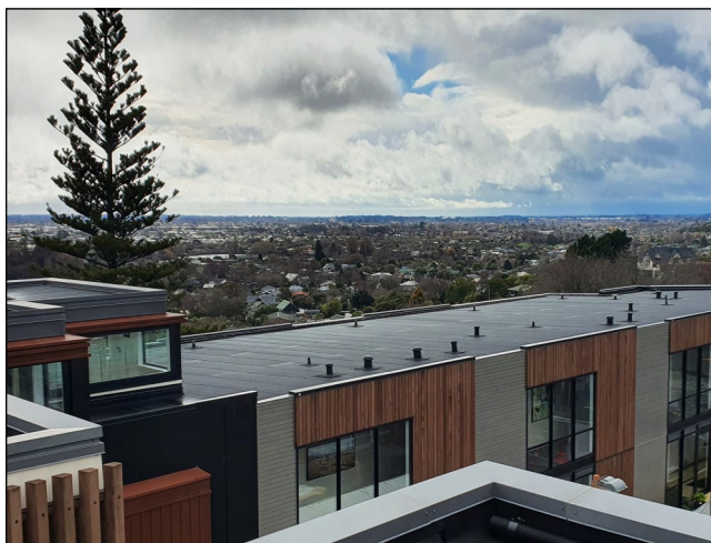
Completed Duotherm warm roof
