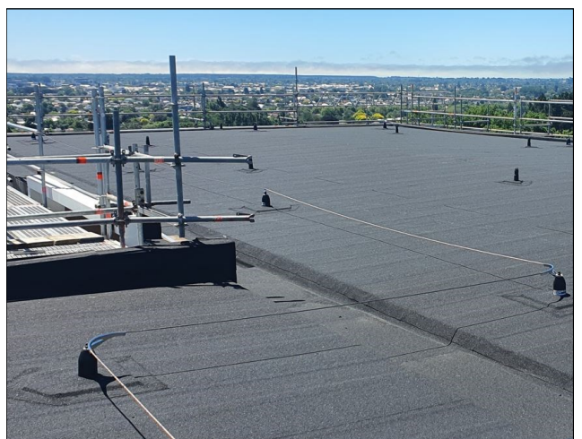
Installation of DuO High Tech waterproofing cap sheet
