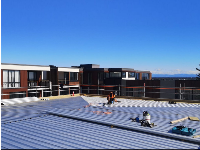
Metal substrate laid to fall
