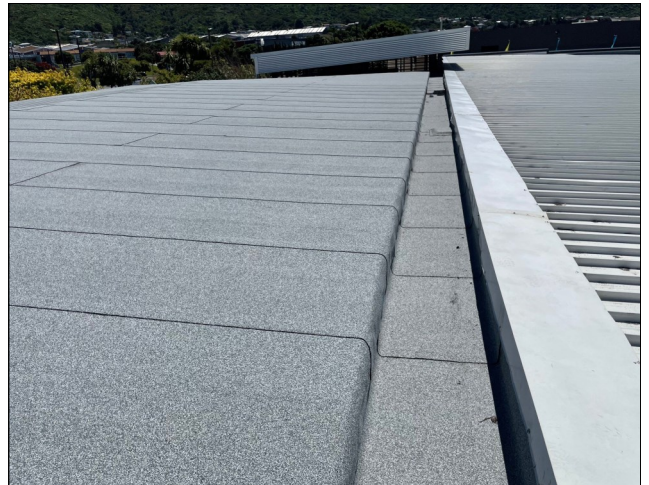
SOPREMA DuO Capsheet Grey/White Installation
