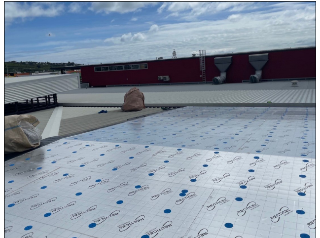
81mm Equus PIR Insulation Installation with Guardian Fastening System
