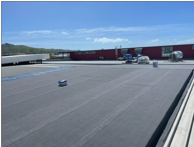
SOPREMA Debotack Aero Basesheet Installation
