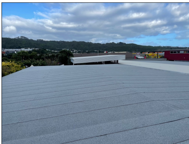
Completed Duotherm Warm Roof
