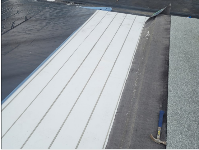
Vapour Barrier over Metal Tray Deck
