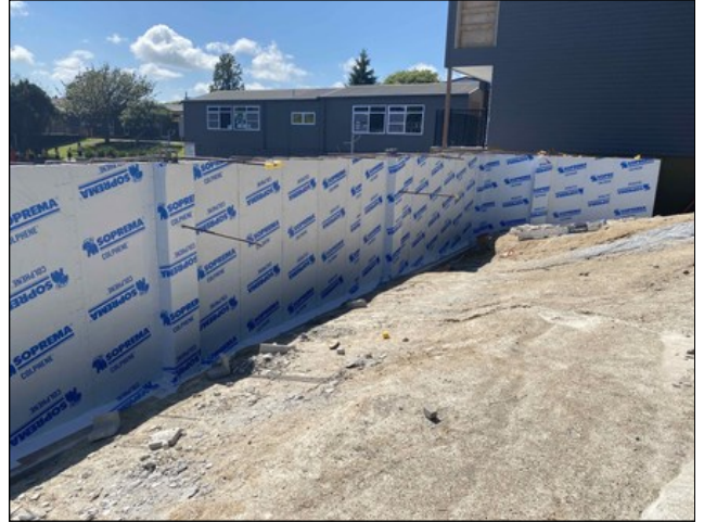
Installation of COLPHENE 3000 below-ground waterproofing
