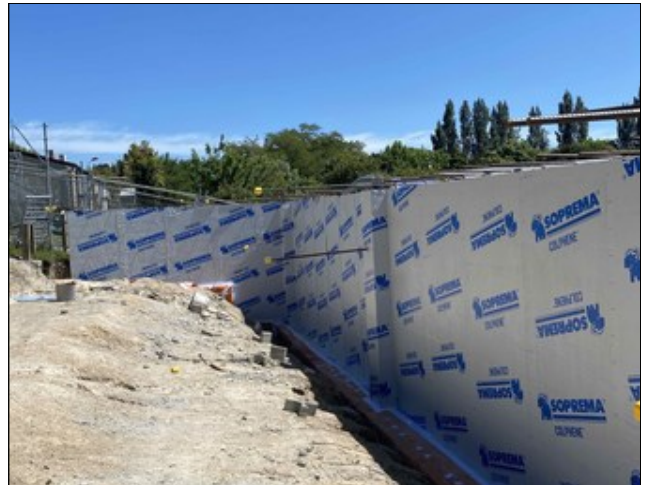
Connection of COLPHENE 3000 waterproofing membrane to DPM
