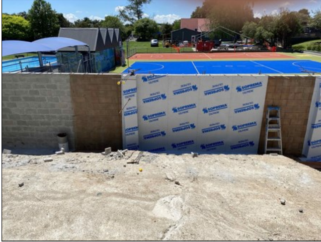
Application of Equus Peel & Stick primer to substrate
