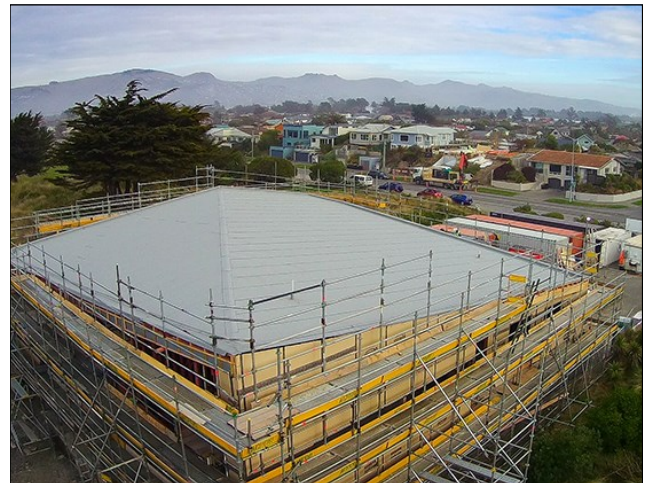
Completed Duotherm warm roof
