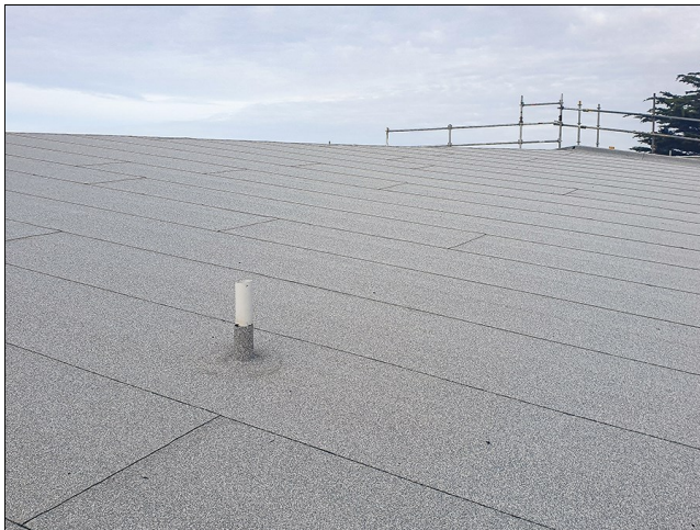
Completed DuO membrane installation
