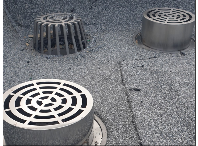
Installation of DuO membrane showing detailing
