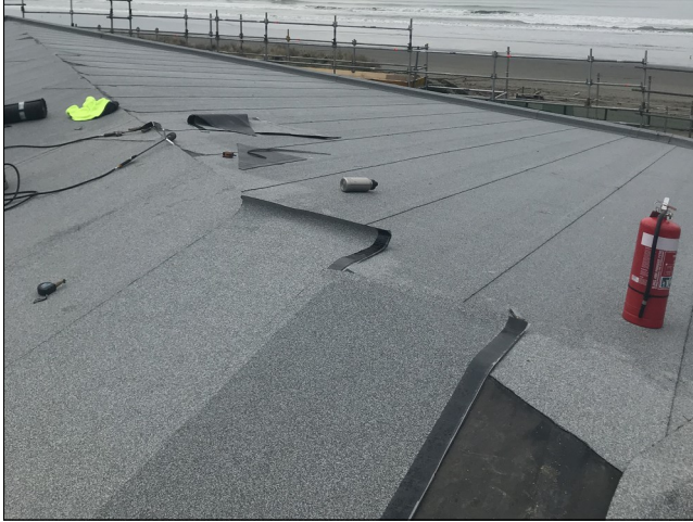
Installation of DuO cap sheet
