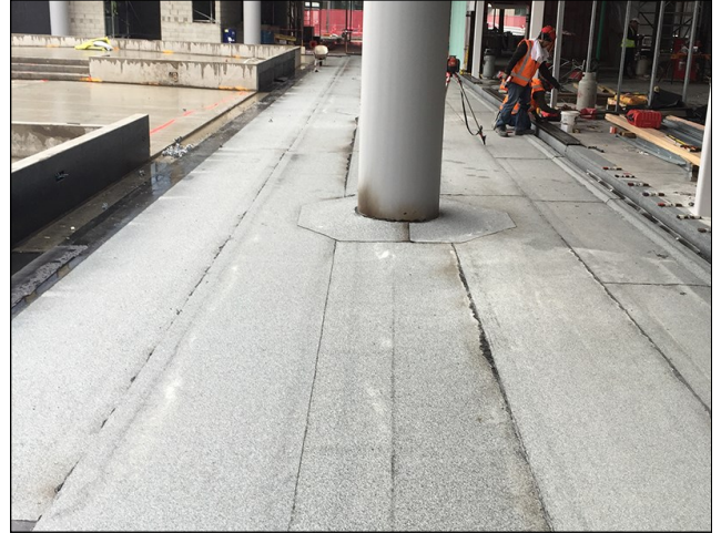
Installation of DuO cap sheet
