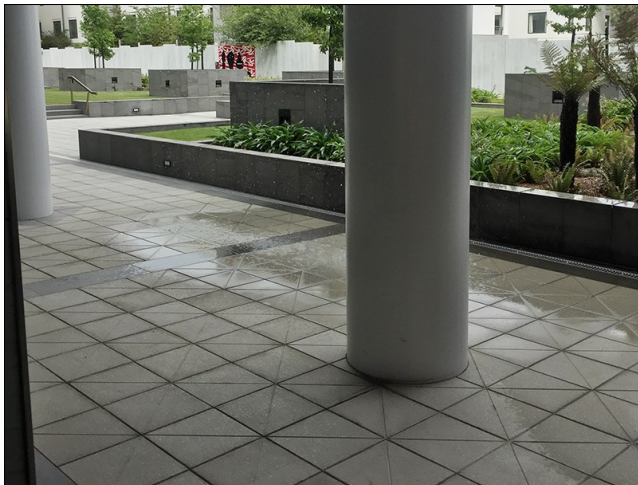
Pavers installed over completed DuO membrane
