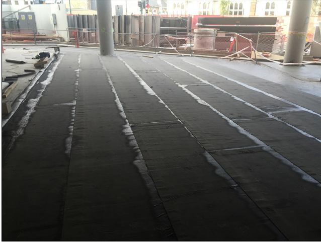
Installation of DuO base sheet over concrete
