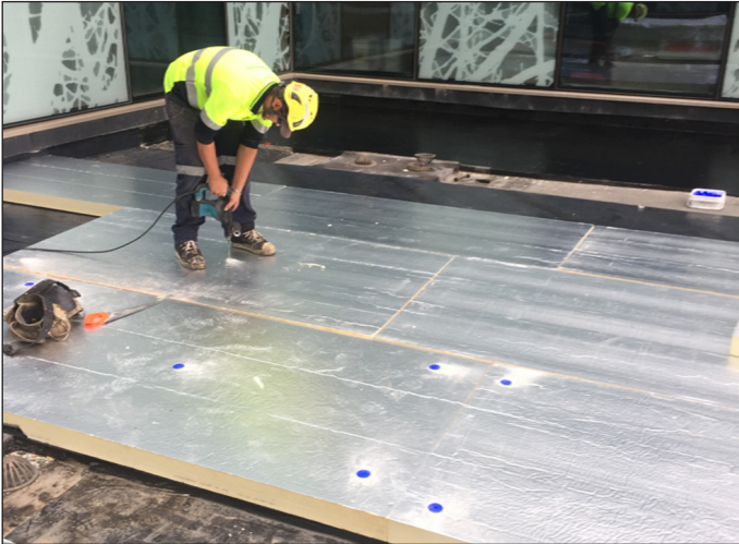
PIR installation over vapour barrier
