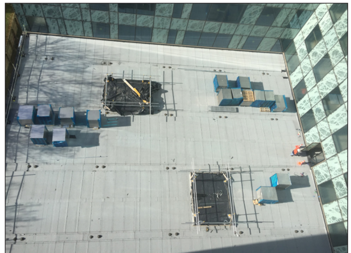
Finished DUOTHERM roof
