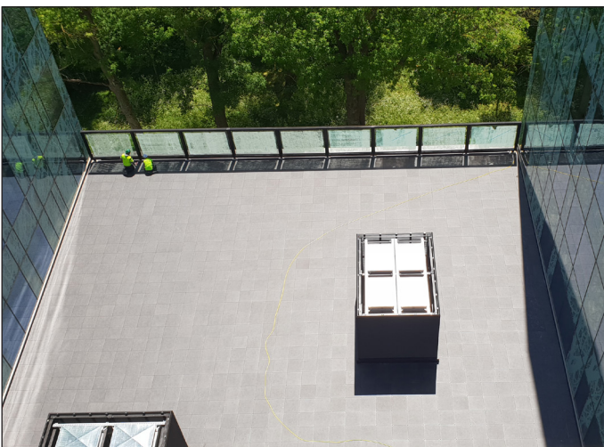
Finished project with pavers
