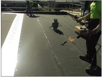
Basesheet mechanically fastened to PIR board
