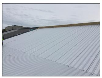
Metal substrate ready for warm roof installation
