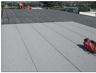
Application of DuO capsheet over basesheet and PIR thermal insulation board
