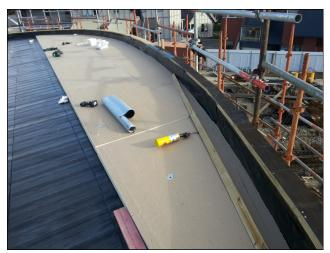
Installation of PIR Board over vapour barrier
