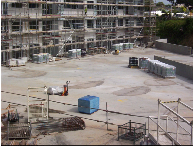
Courtyard site preparation
