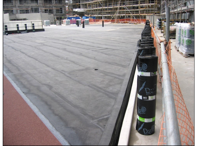
Basesheet membrane applicaion
