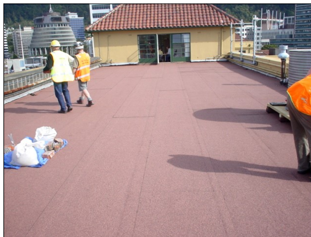
Completed roof refurbishment
