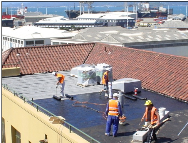
Preparation of area, primer and basesheet application
