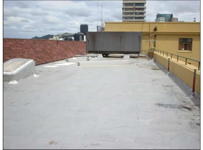
Existing roof before renovation
