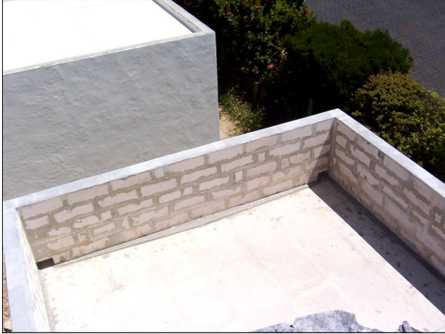
Hebel block structure
