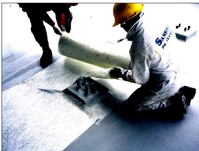
Fibreglass detailing
