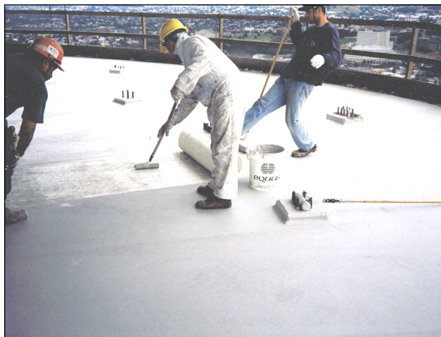
Fibreglass reinforcement installed into wet Dexx body coat
