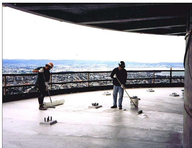
Chevaline Dexx application over fibreglass
