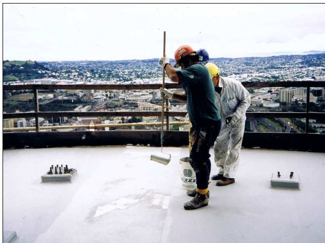
Priming concrete substrate
