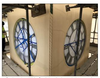
Crack repair and Keim Granital application to clock tower walls
