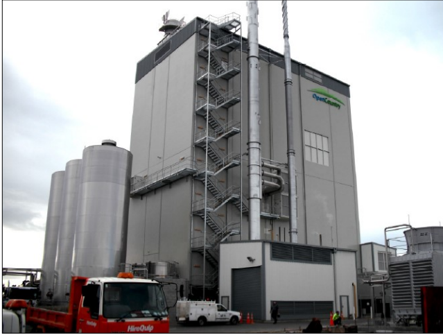
Chevaline Colouglaze to exterior concrete
