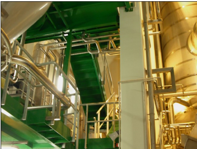
Colourcure to steelwork
