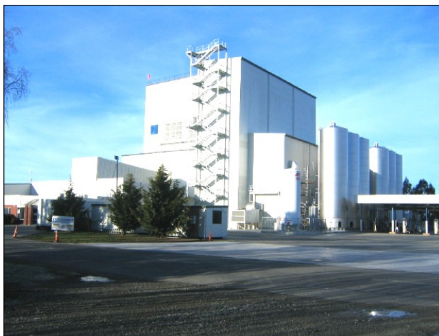
Chevaline Colourglaze to exterior walls
