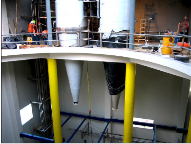
Chevaline Colourglaze to interior walls
