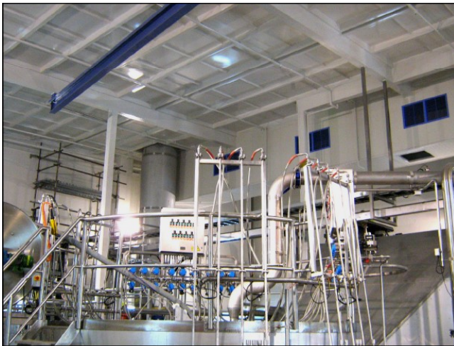
Steel roof structure
