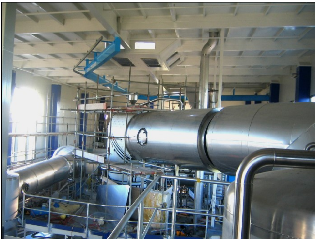
Steel roof structure
