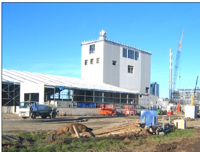
Chevaline Colourglaze to exterior walls
