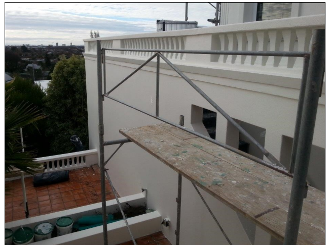
Troweltexx 2000 plaster applied and painted
