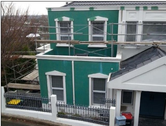
Detail Plaster applied to entire building
