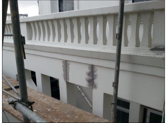
Crack repairs
